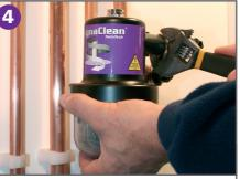
Loosely secure the MagnaClean TwinTech canister to the valves, following the flow direction indicated on the canister. Tighten the compression fittings, being careful not to over tighten.
