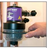
Re-attach the clear base to the top section of MagnaClean TwinTech and tighten until sealed. Do not over tighten.
