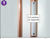
Drain the central heating system or plug-off feed and expansion tank and release the system pressure. Measure and mark an appropriate section when making the connections with elbows as shown (Refer to the Installation Instructions inside the box). When installing above a boiler or other object allow 95mm clearance between the magnet cap to the top of the boiler or other object for the removal of the clear base when servicing.
