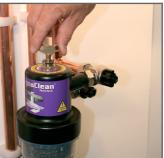
Open the isolation valves to the marked ON position and vent through the Pro-Fill air vent. When venting, protect the surface below the canister with the servicing tray provided to capture any drops of water. Run the central heating system while checking for leaks. Repeat steps 1 - 6 if required. Ensure the filter is thoroughly clean before leaving the premises.
