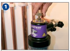
With a standard radiator key, remove the Pro-Fill air vent. The built-in, one-way valve will prevent water from escaping. Attach the chemical adapter and feed in the chemical.
