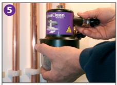
Loosen off the valve flange nuts and insert the rubber washers provided. Tighten the flange nuts. Do not over tighten. Refill the heating system.
