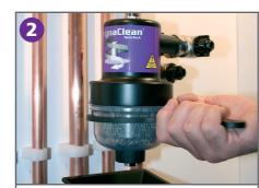
Loosen the canister base with the large spanner while holding the tray beneath. Carefully unscrew the clear base. Allow water to collect in the servicing tray supplied.
