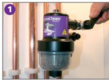
Important - Before commencing any servicing work turn off the electrical supply to the boiler. Turn both isolation valves to the marked OFF position. Loosen the air vent to release internal pressure. When venting, protect the surface below the canister with the servicing tray provided to capture any drops of water.
