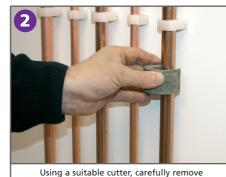
the marked section of pipework to create the correct opening.
